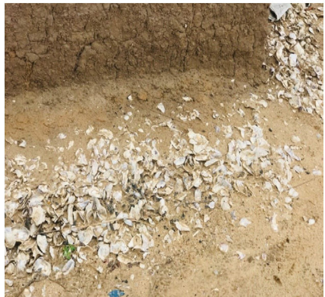
PHOTO 21: OYSTER SHELLS AS PART OF THE FOUNDATION OF A MUD HOUSE AT GBLIKPE
